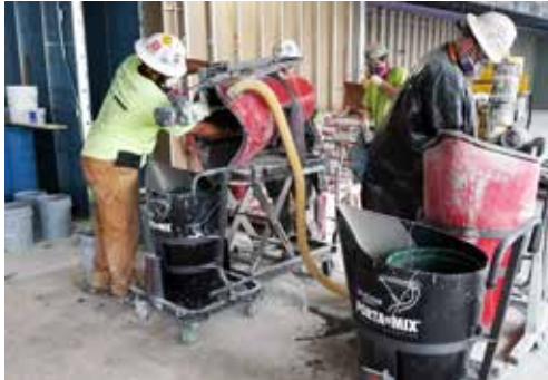
TRU® Self-Leveling – Mixing with a strainer
