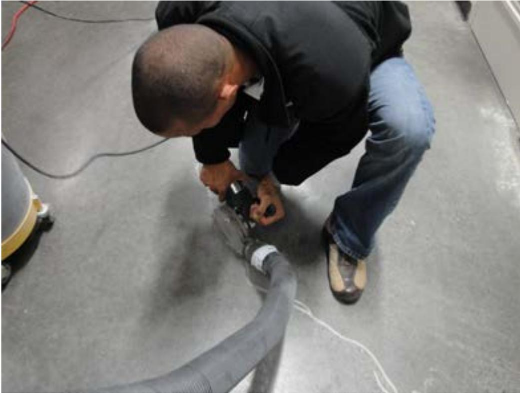
*Step 1: Chase cracks using vacuum equipped angle grinder with diamond blade to a nominal depth of 1/2".*
