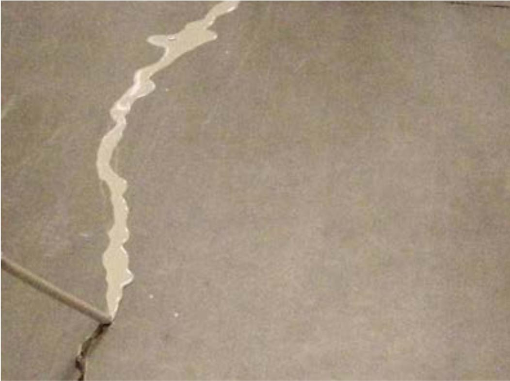
*Step 2: Gradually overfill crack with Spal-Pro RS 88. Monitor for seepage and refill as needed prior to material cure.*
