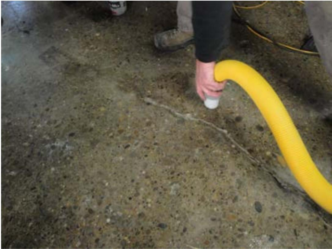
*Step 2: Vacuum clean, ensuring crack is free of all loose debris and dust.*
