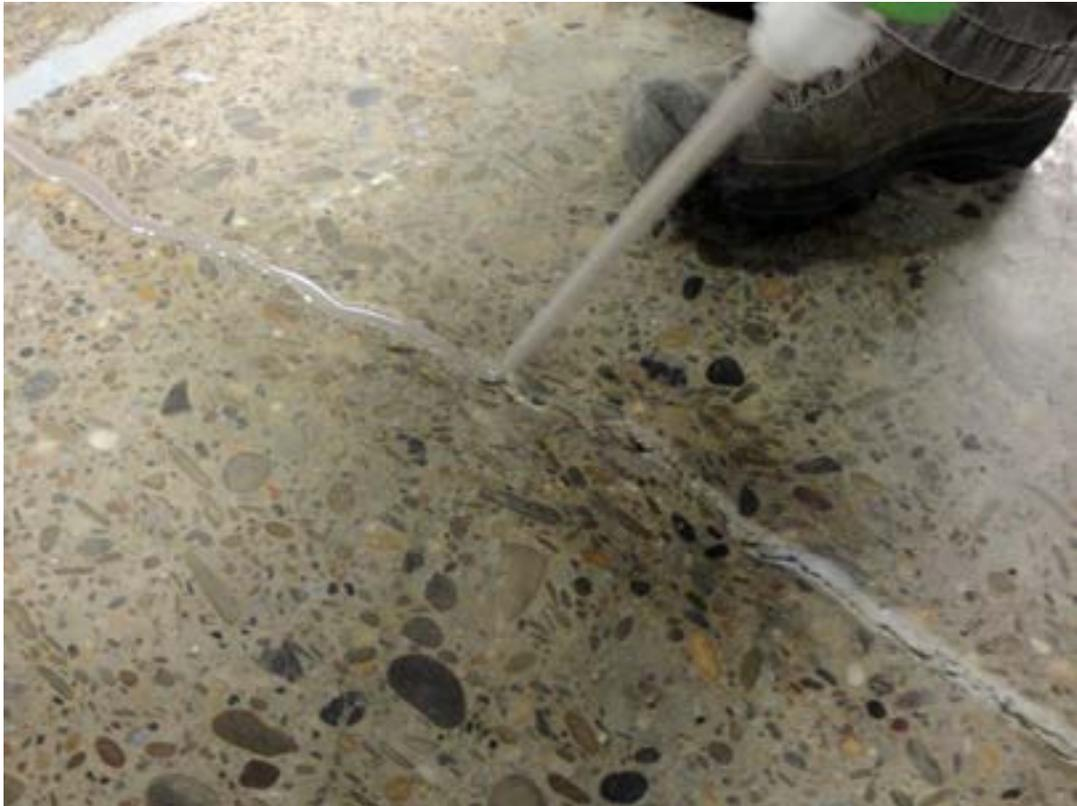
*Step 3: Gradually overfill crack with Rapid Refloor.
