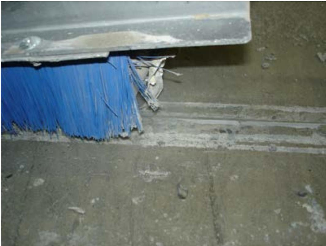
*Step 1: Saw cut lines behind outside of joint spalling to a nominal depth of 3/4"*
