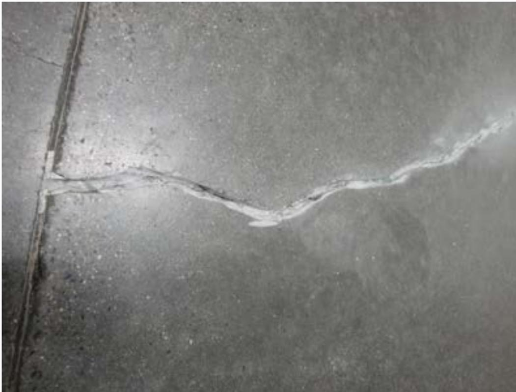
*Example of properly prepared crack. Edges should be neat and crisp; nominal depth of repair 1/2" deep.*
