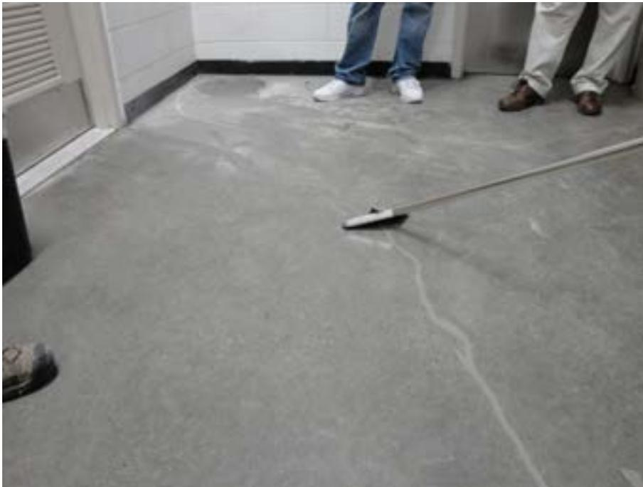
*Step 3: After Spal-Pro RS 88 cures (approximately 45 minutes minimum) razor off overfill leaving flush filler profile. Monitor various razoring times to find best finished profile.*
