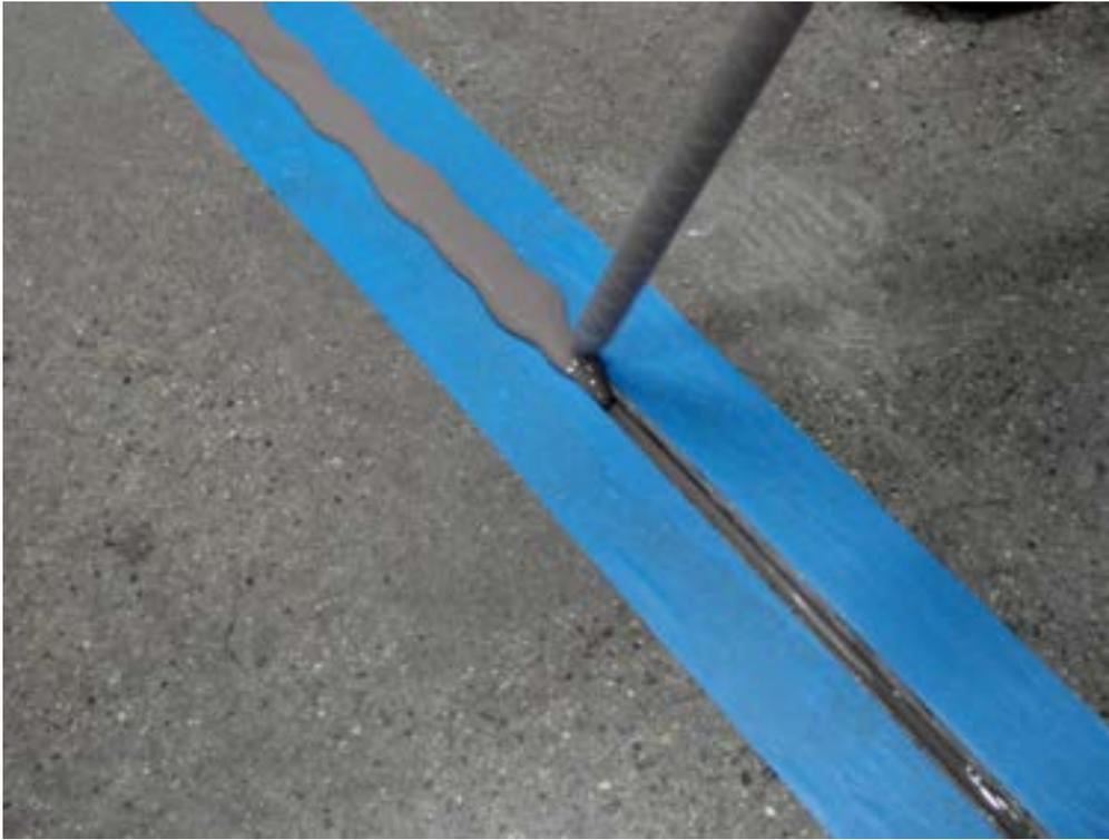
*Step 2: Protect slab surface along joints using removable tape or Metzger/McGuire's SPF-P (stain prevention film). Slightly overfill joint with Spal-Pro RS 88 (color to match adjacent surface). Monitor regularly for seepage and re-apply if needed.*
