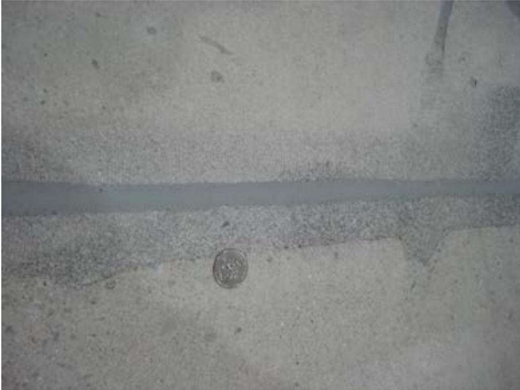
*Step 9: Razor off Spal-Pro RS 88 overfill flush with repair/floor surface.*
