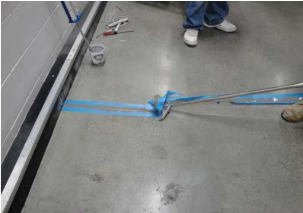
*Step 3: After cure razor off excess using razor scraper equipped with disposable blades.
