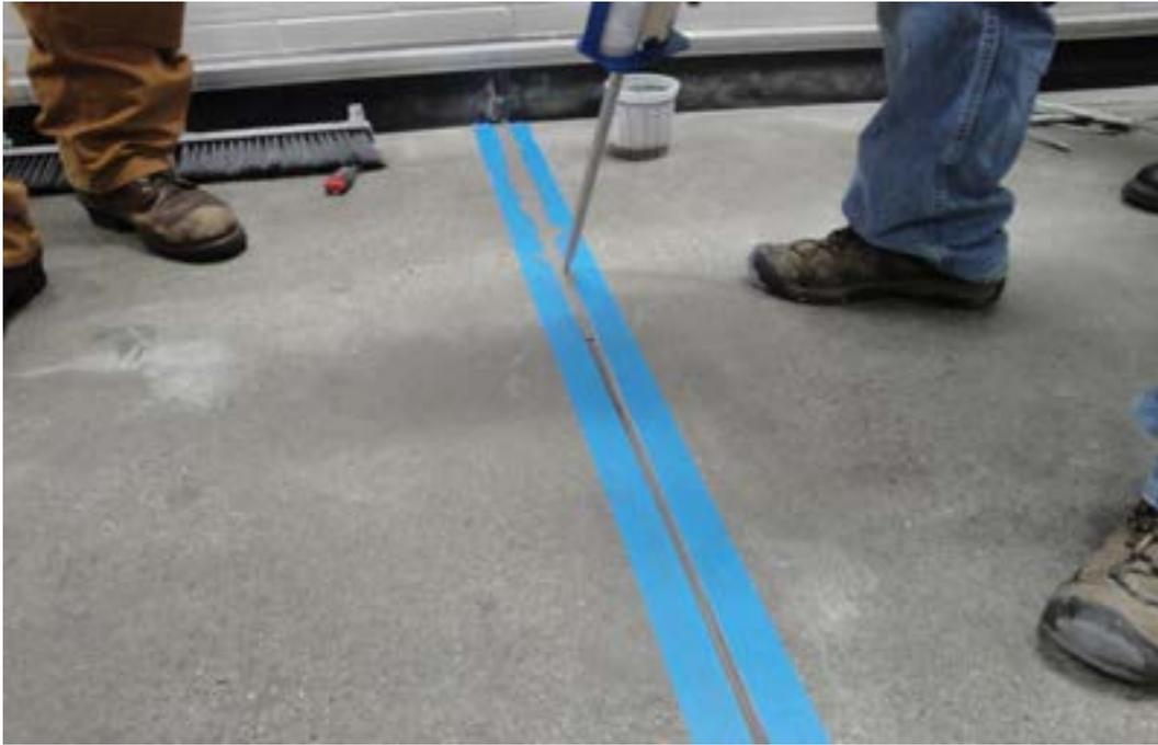
*Step 2: Slightly overfill joint with Spal-Pro RS 88.
