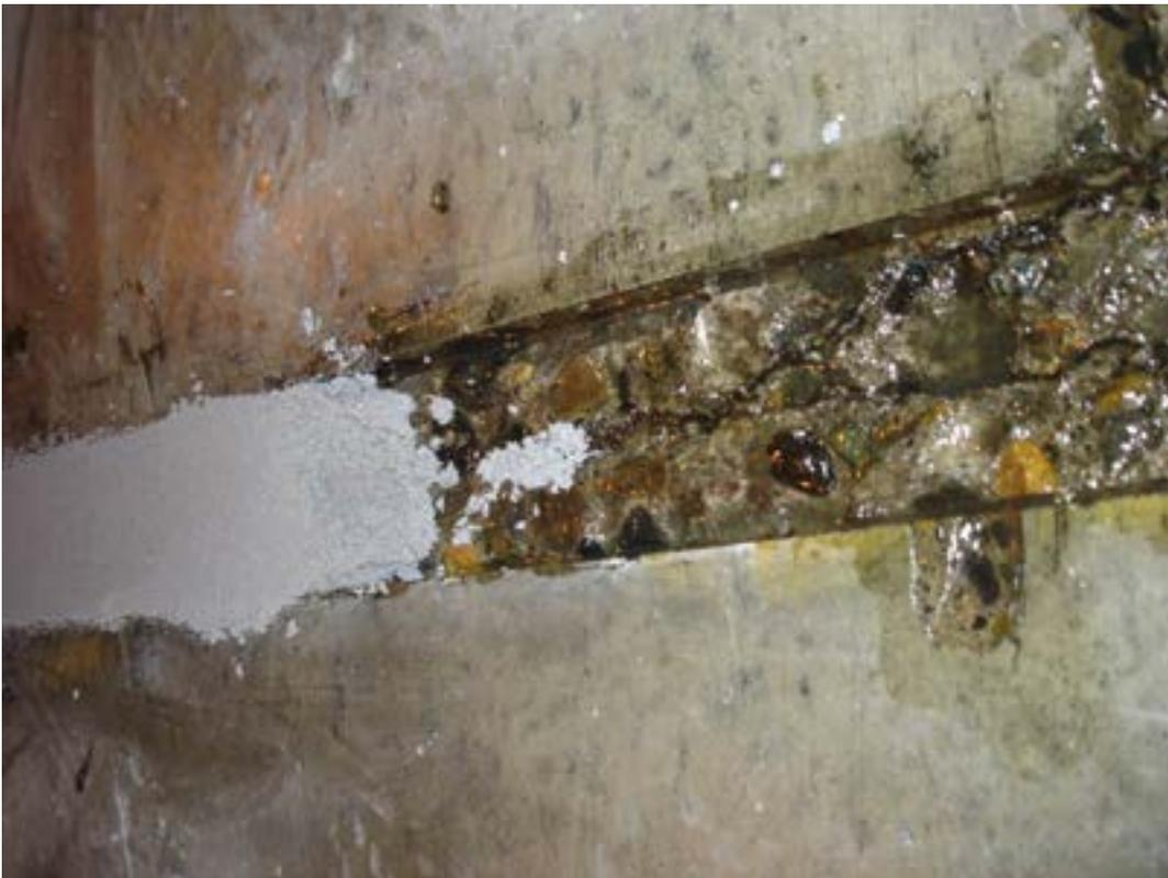
*Step 3: Fill channel with Armor Hard Extreme mortar, trowel flush with floor surface*
