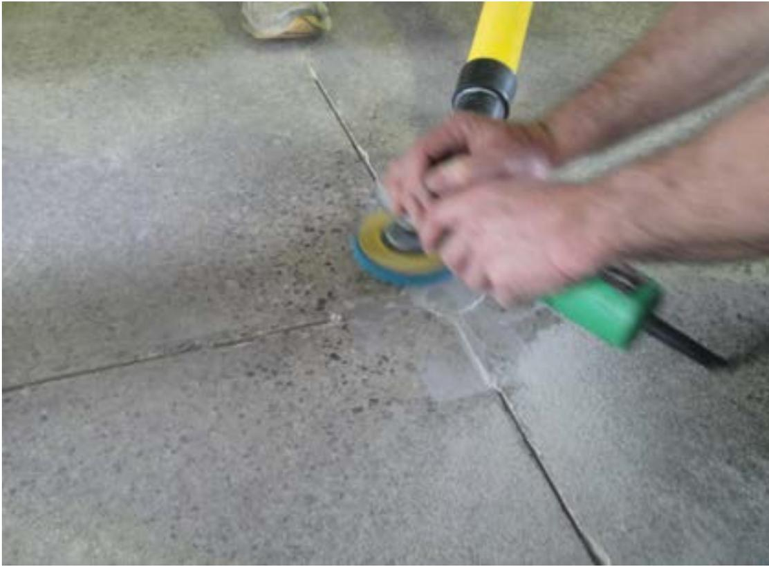
*Step 2: Grind off Rapid Refloor overfill flush with floor surface.*
