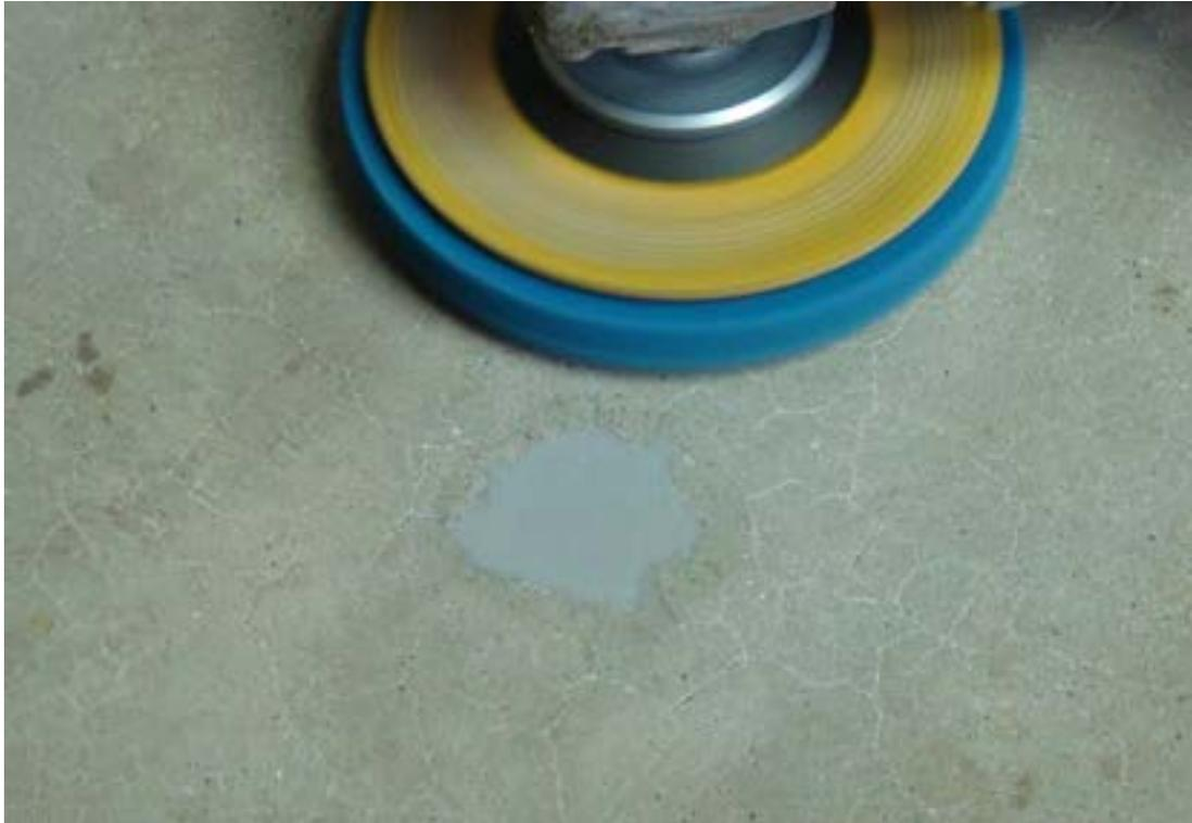
*Step 3: Grind off cured material flush with floor surface.*
